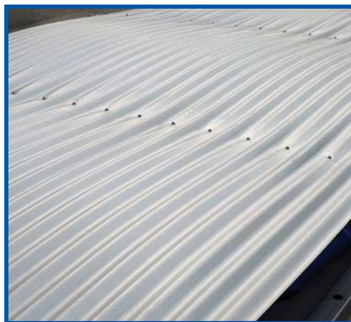
Roof Pressure Test
