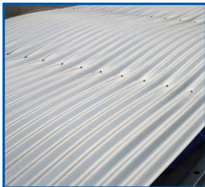
Roof Pressure Test
