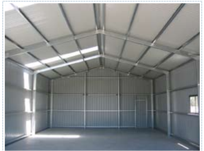
SKYLIGHTS, MANDOOR & WINDOWS
