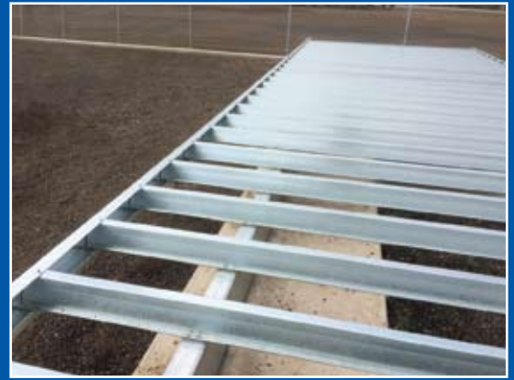
Just set the foundations in concrete.
