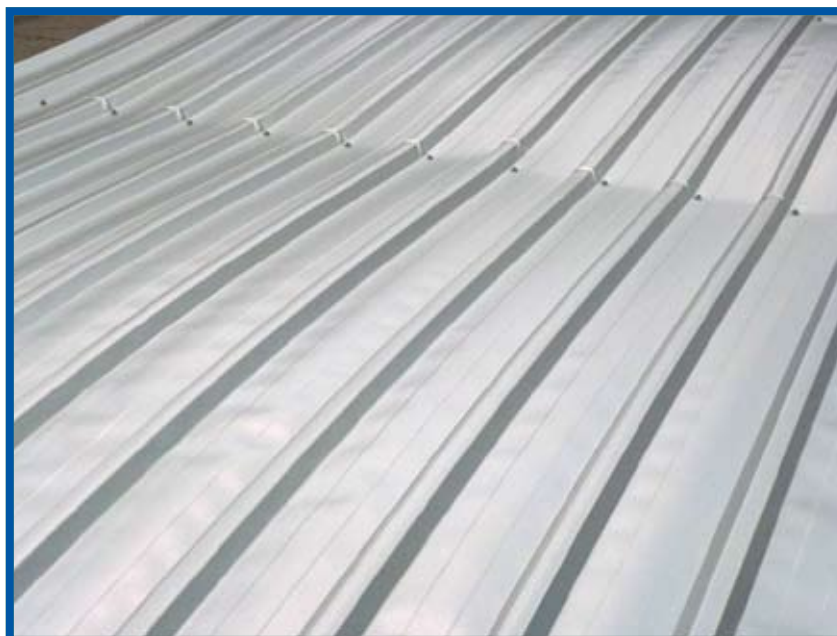
Roof Pressure Test
